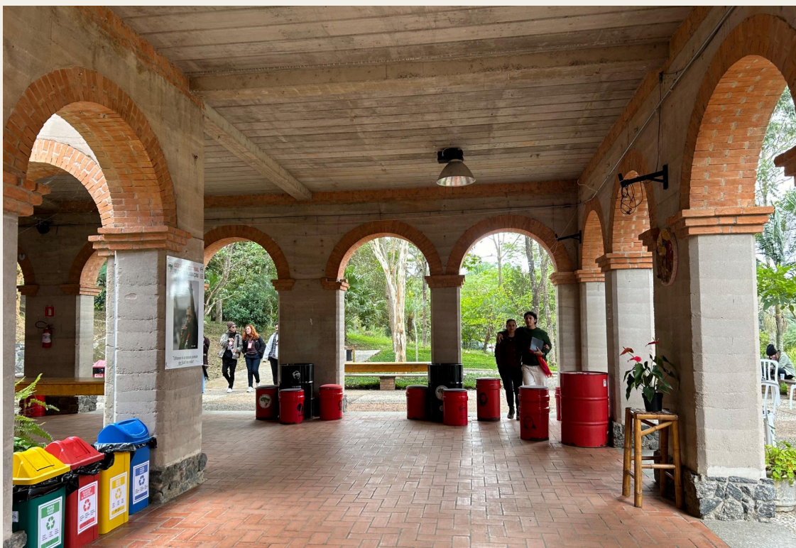
Lower area of the refectory: rammed earth and BTC columns. Photo: Cecília Santos, 2024.
