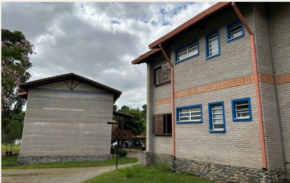
Detail of the walls of the accommodation and their stone bases. Photo: Cecília Santos, 2024.
